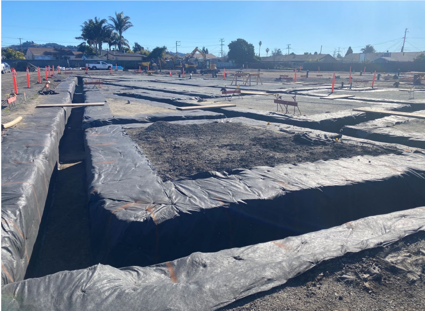
Protected Excavations of Building Footings and Utility Trenches
