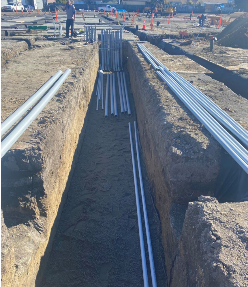
Underground Electrical Conduit Installation Before and After
