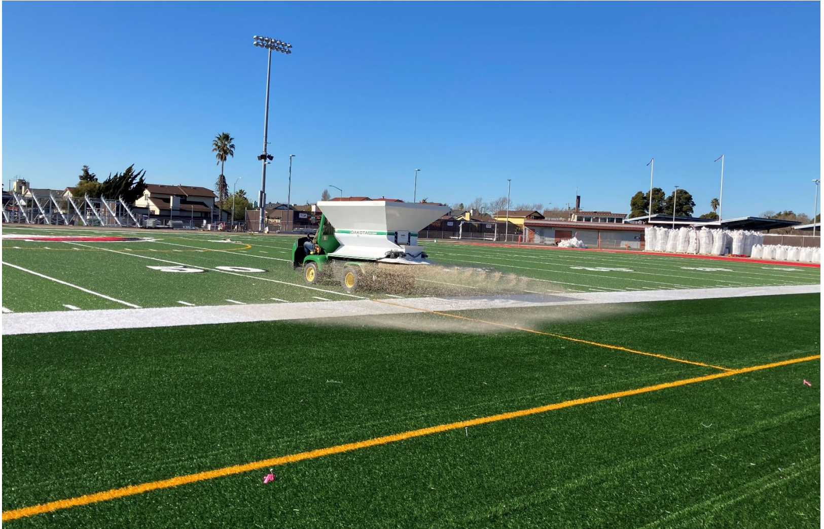
Installed Field Surface with Infill being Dispersed
