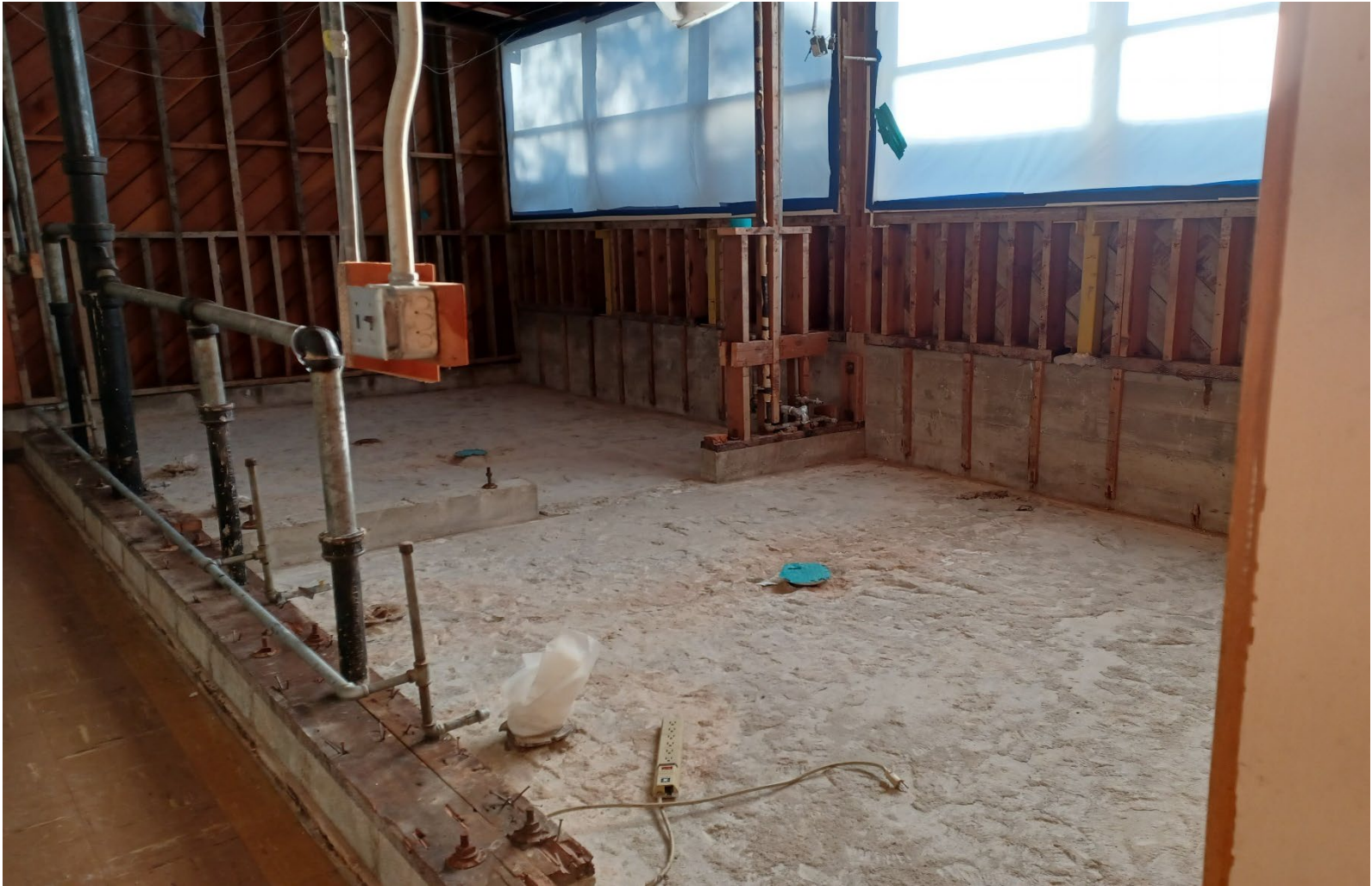
Selective Interior Demolition Ongoing
